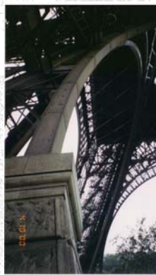
Figure 103: Base Detail, Eiffel Tower
