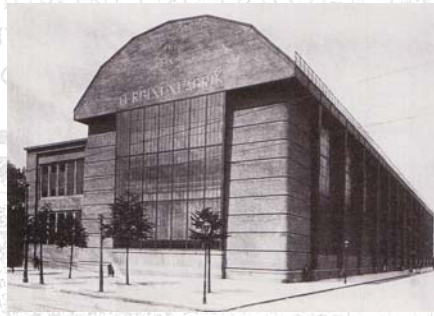
Figure 135: AEG Turbine Plant (1909)
