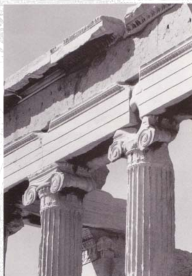
Figure 5: Grecian Column Detail
