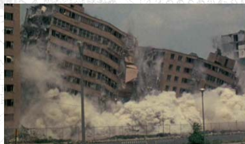
Figure 149: The Demolition Scene
