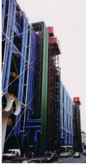
Figure 159: Pompidou Centre, Paris (1972)
