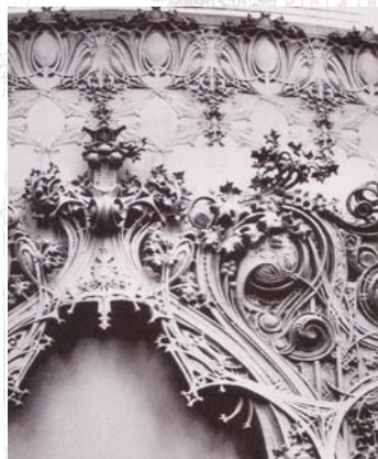
Figure 122: Wrought Iron Detail, CPS Store (1899)
