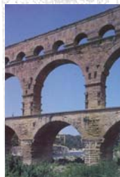
Figure 29: Aqueduct, Nimes, France (50 a.d.)
