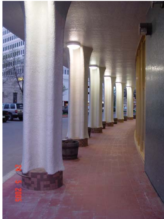
Figure 44: Exterior Columns, SaskPower Building (J. Pettick Architect)
