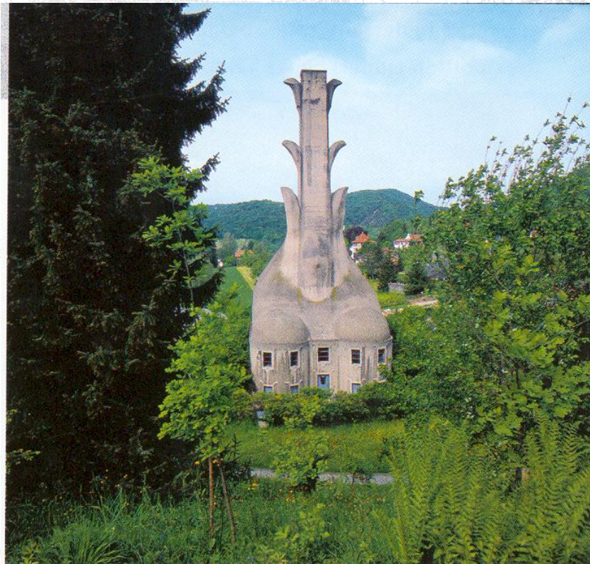
Figure 3: Goetheanum Boiler House, Dornach, Switzerland
